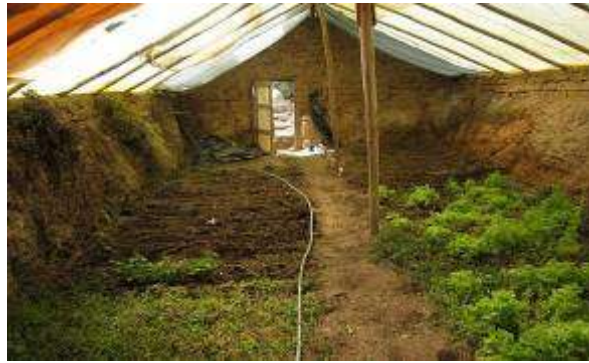
Figure 1 Internal of an earth sheltered greenhouse [10]
